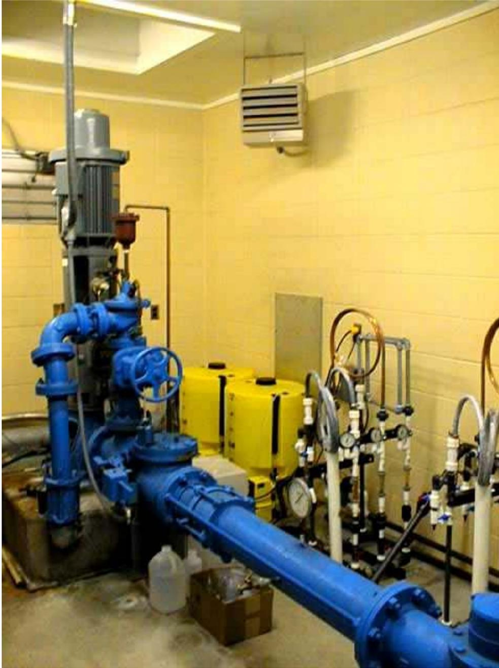
*A close up view of a pipe loop rack at the Village of Lone Rock. The pipe above the floor drain discharges the apparatus' water. The rectangular box on the wall is the controlling timer. (The water on the floor comes from a dehumidifier in the left hand corner of the picture.)*
