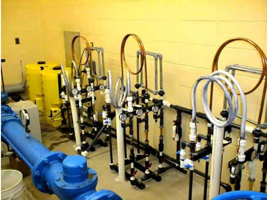
*Pipe loop apparatus at the Village of Lone Rock Well No. 2 pump house. The loop racks extend along the side wall of the pump house. In the back corner are chemical tanks and pumps for sodium hydroxide and sodium hypochlorite.*
